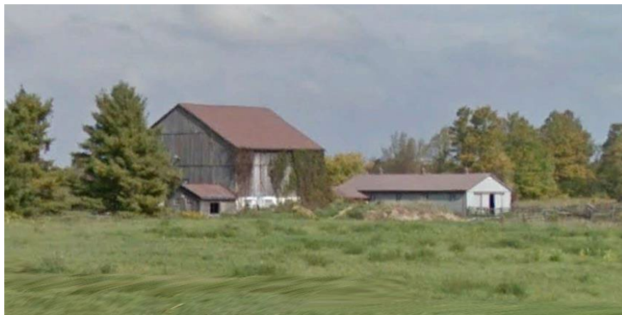
Barn and shed located at #17757 Shaws Creek Road (Source: Google Earth)
