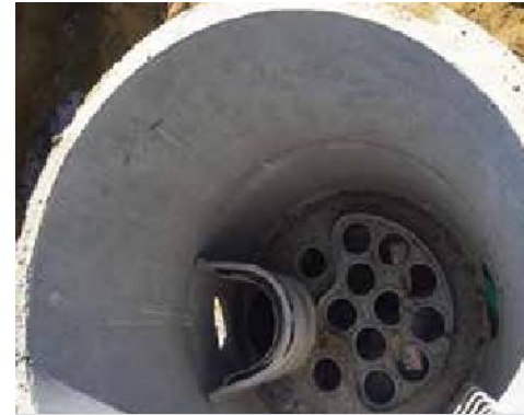
Provided technical support at installation
